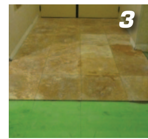
3 Lay Thinset and Flooring Directly on GreenSkin™
