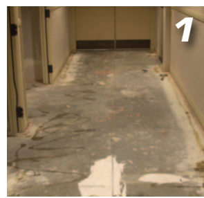
1 Wet Mop Clean to Prepare Surface (No Need to Prime)
